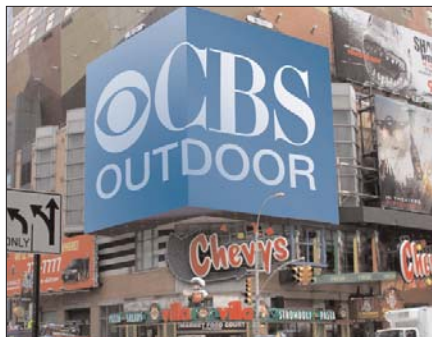
Times Square Cube under construction
