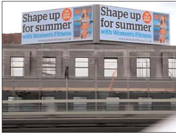
The CBS OUTDOOR Site 76 digital billboard on the UK's the high traffic M4 motorway.
